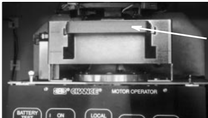
Photo B Shift handle in COUPLED position
